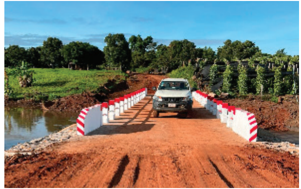
River Crossing, Mondulkiri (Credit: Socfin Cambodia, 2022)
